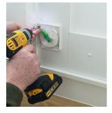
1. Screw the Squebble base plate unit in the correct dwelling location next to active kit with a working power socket within 1 metre (make a note of where the cable exit needs to be).
