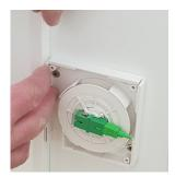
3. Unwind the 'long end' of the fibre from the internal cartridge and place alongside the Cable route which has been cleaned to the exit hole.
